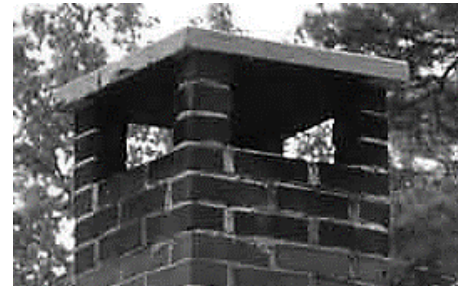
Concrete Cap Chimney Top
